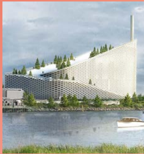
© Amager Bakke / Copenhill
